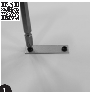
1 Fix steel plates with suitable screws (min. 4 steel plates per metre/40").
